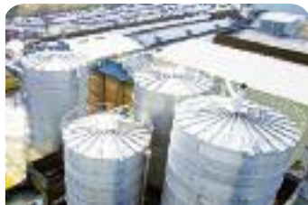
The new stock preparation plant was a major part of the investment to modify New Thames Mill at Kemsley.
